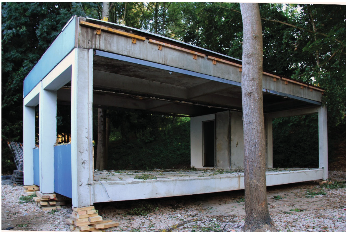
Fig.1 In 2016, two modules of the former student village at the VUB campus were stripped and -as a way of experiment- picked up and dropped off at the other side of the campus – © Waldo Galle, VUB Architectural Engineering.
