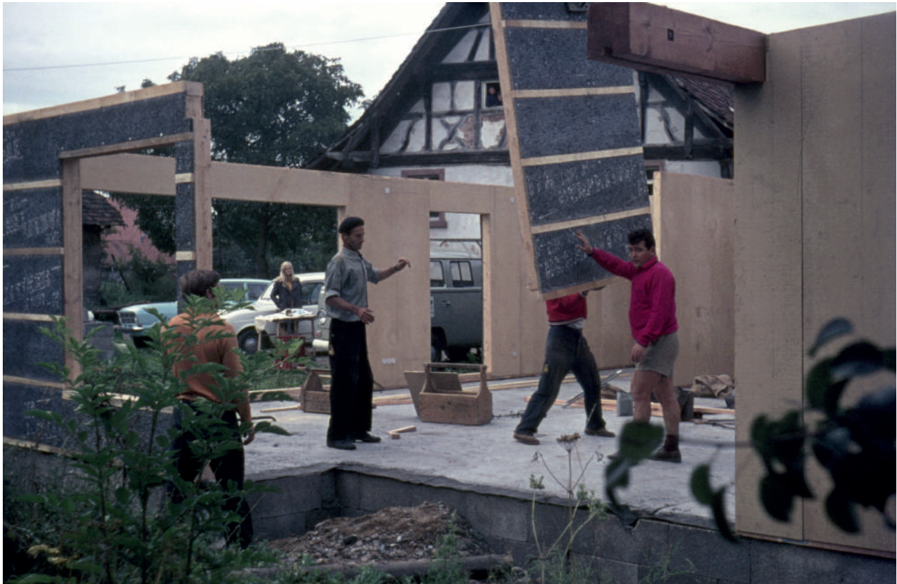
[2] Assembly of the prefab kit, 1971. Photo: Peter Pietsch.
