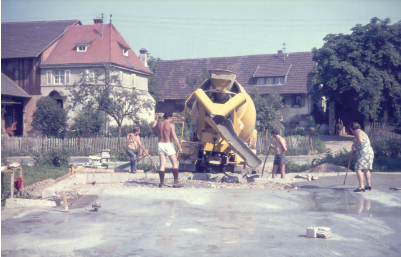
[1] Pouring of the floor slab, 1971. Photo: Antje Pietsch.
