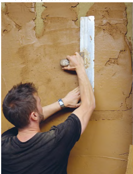
BBB PG hands on explorations: earthen plaster
