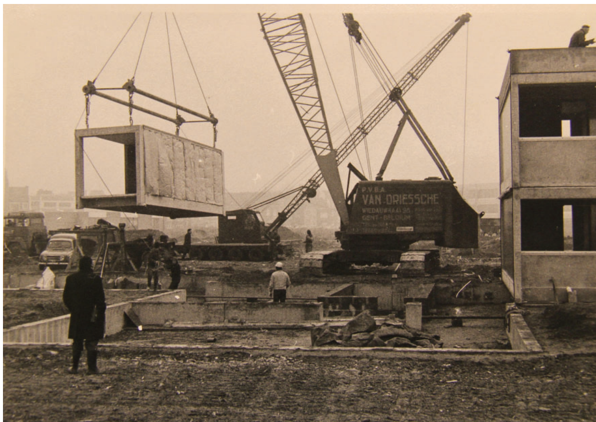
Fig.2 Delivery of the modular units for the construction of the student homes at the VUB campus in Elsene in 1973 – © Archive of the Technical Service 'Infra' of the Vrije Universiteit Brussel.
